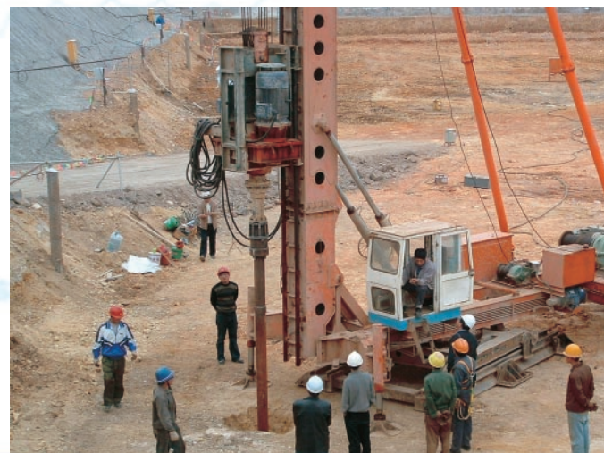
(Right) Electric rig installing screw piles
