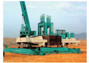
(Above) Static piling rig
