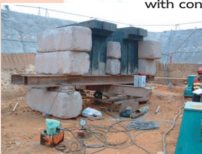
(Left) Testing piles
